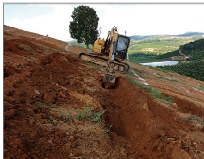
Figure 10. Furrows pening in sloping areas using the backhoe. Marking lines using limestone.
