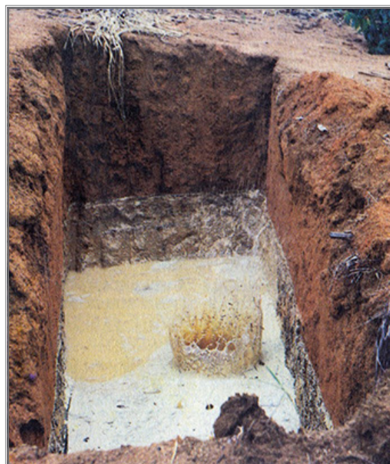
Figure 12. Dry box constructed in the internal area of the crop to reduce the superficial flow and capture rainwater.
